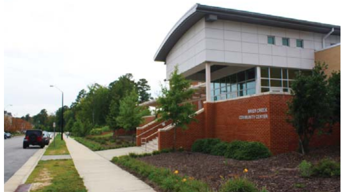
Brier Creek Community Center
