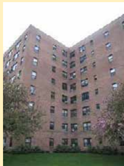
More than a third of New Rochelle's households are in multiple dwelling units like this one on Pelham Road.
