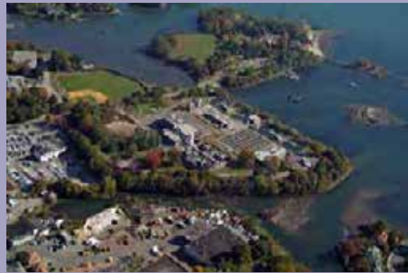
The New Rochelle Sewage Treatment Plant is being upgraded to a treatment capacity of 20.6 million gallons per day.
