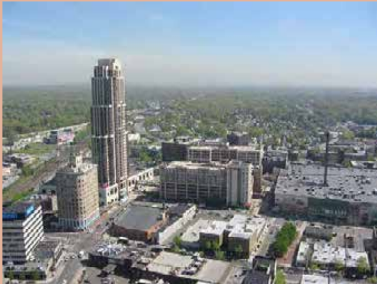
New Rochelle's downtown has multiple access points, but many feature poor function or design.
