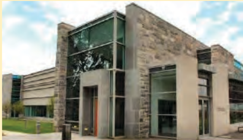
The new Wellness Center at the College of New Rochelle incorporates many green design features.
