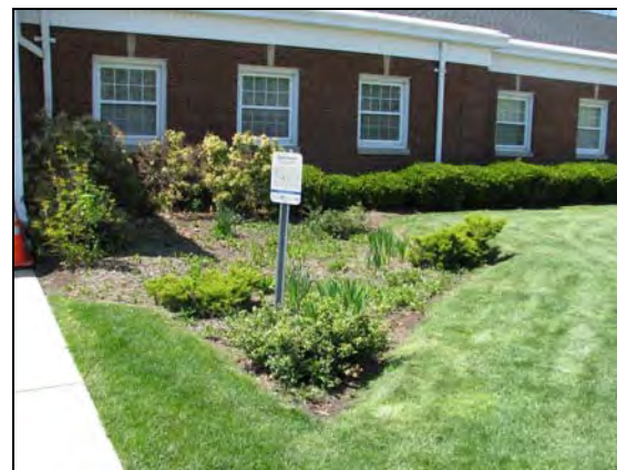
Rain Garden Installation, Parsippany- Troy Hills Township Municipal Building
