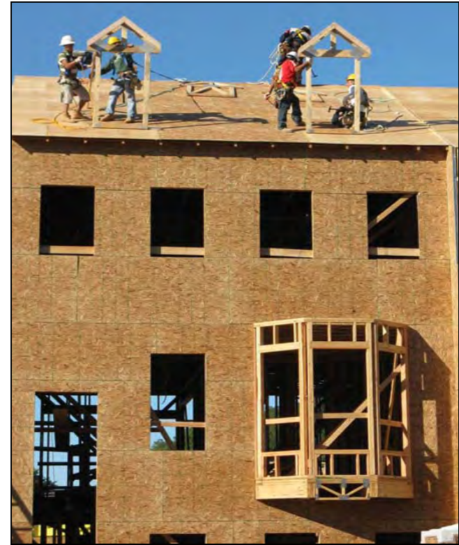
Construction of Morristown Square townhomes, Morristown.
