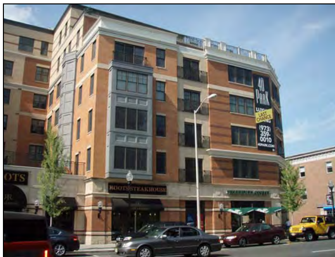
40 Park Luxury Condominiums, Morristown (Redeveloped site of the former Epsteins Department Store)
