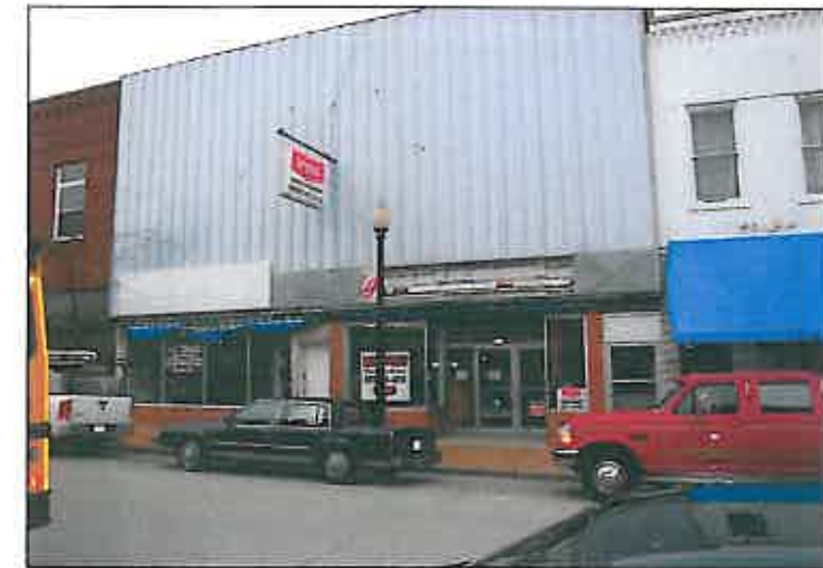
Existing vacant retail space opportunity in Downtown Mexico.
