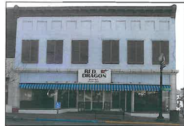
The former JC Penny building located on the Village Square.
