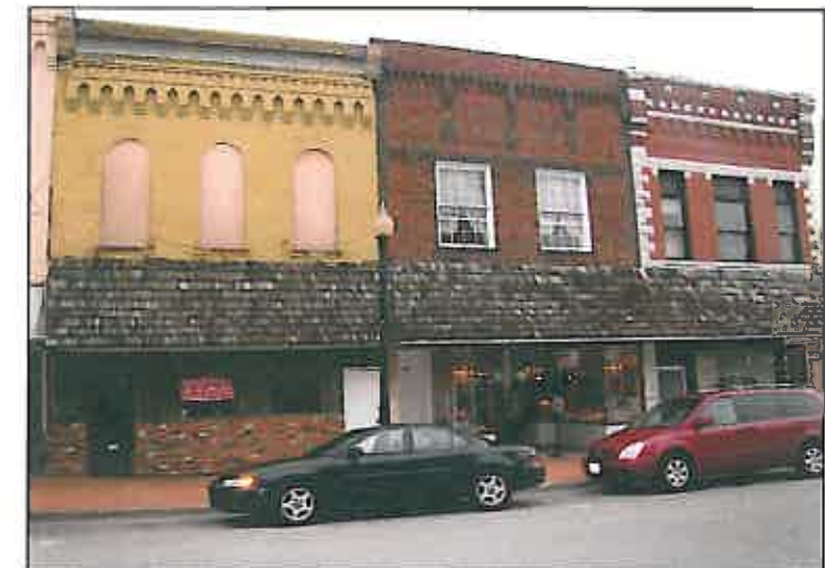
Funding can also be used for awning removal where desired in Downtown Mexico.
