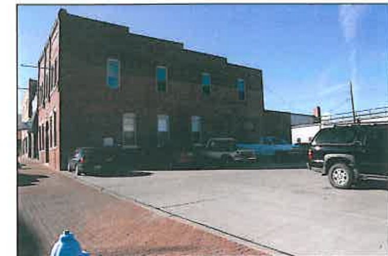
TIF funds could be used to enhance and expand public parking lots to accommodate Downtown visitors/employees.
