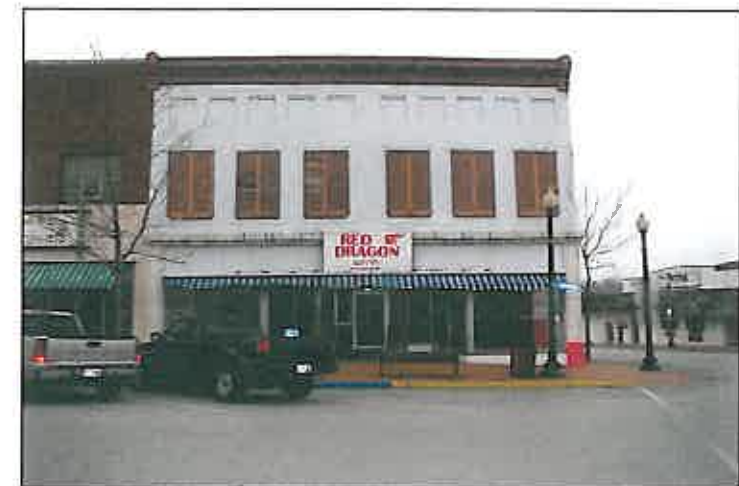
Existing vacant retail space opportunity in Downtown Mexico.
