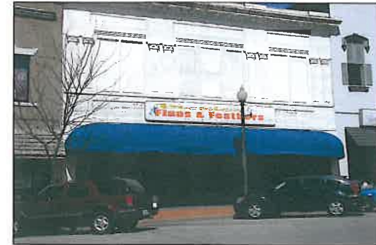
Existing vacant retail space opportunity in Downtown Mexico.
