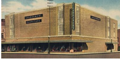
Landkamer Building > formerly the Landkamer Furniture Store (photo: flickr.com/photos )
