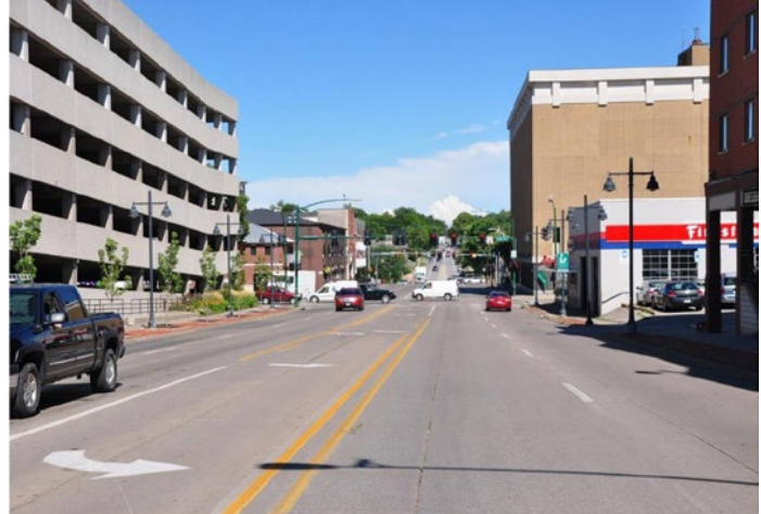
Existing conditions Burlington Street
