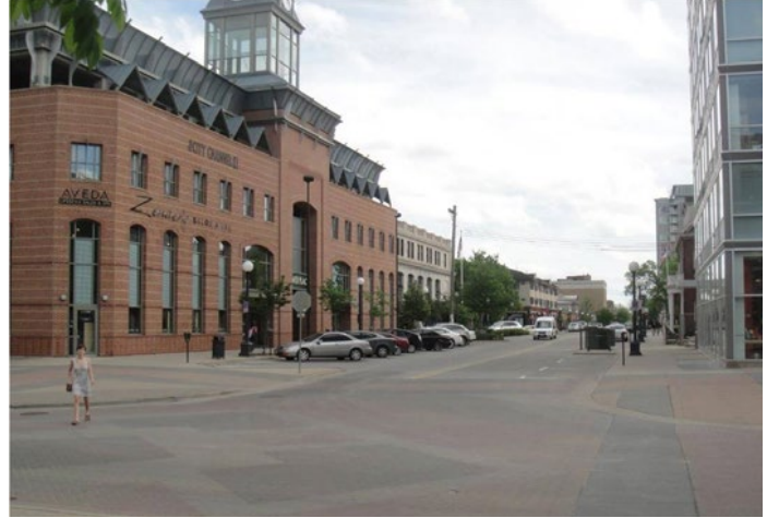
Existing conditions Linn Street
