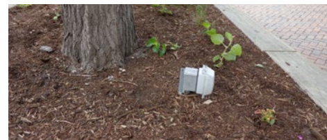
Existing electrical outlet in planting area
