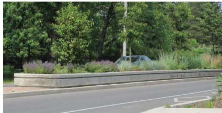
Raised median planters could be constructed along East Main Street where turn lanes are not needed east of Cronkhite Avenue
