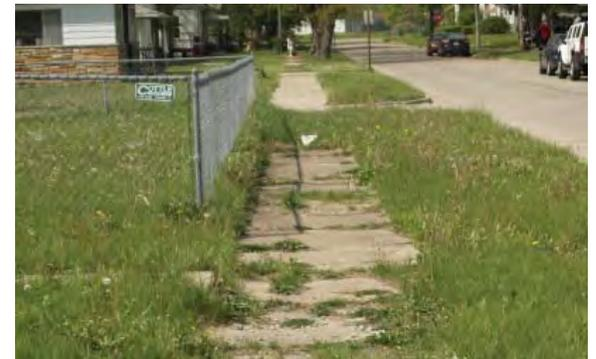
*Some blocks appear to have “disappearing sidewalks” where weeds and lawn have begun to grow over failing concrete*
