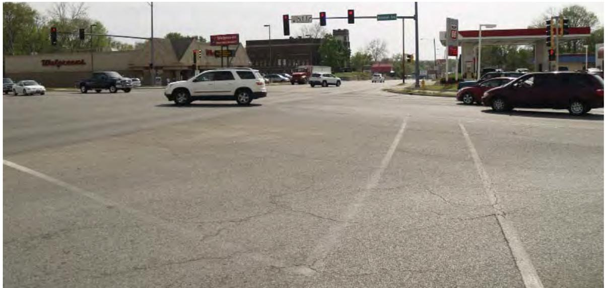
*Crosswalks are marked in all four directions at the signalized intersections, however some crosswalks have begun to fade*
