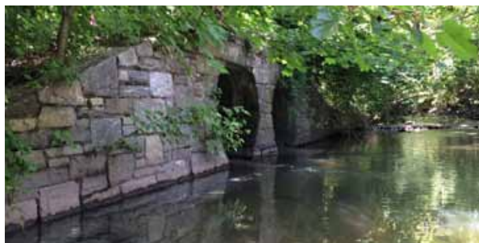
A location for stormwater discharge in Mount Vernon
