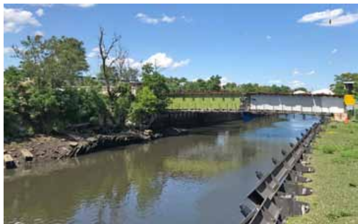
The Fulton Avenue drawbridge is currently under construction and closed, blocking any water borne traffic further north. The edges of the canal vary in condition. Many of the edges along the Mount Vernon side (left) need reinforcement.
