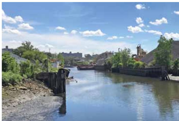
The metal sea walls show the change in water level due to the tides. Here at low tide you start to see the edges of the bottom of the canal. Looking south, you can see a barge servicing the asphalt plant.
