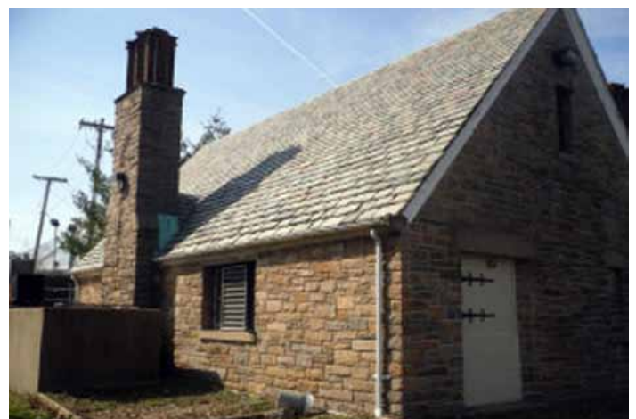
Hutchinson Pump Station
