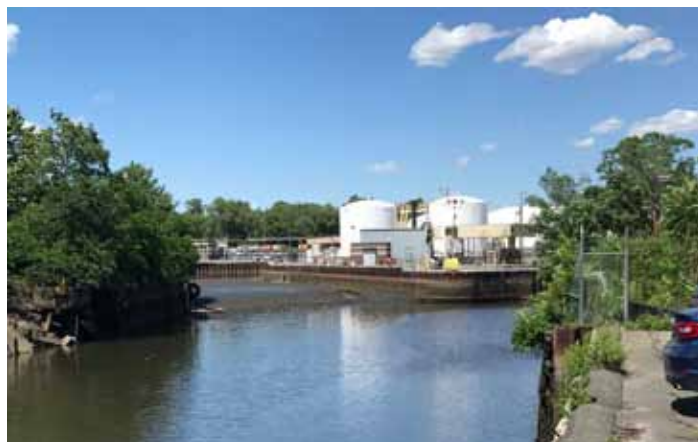
The buildup of silt is quite visible at the "Y" of the canal north of the Fulton Avenue bridge. This could be the spoils pile from previous dredging
