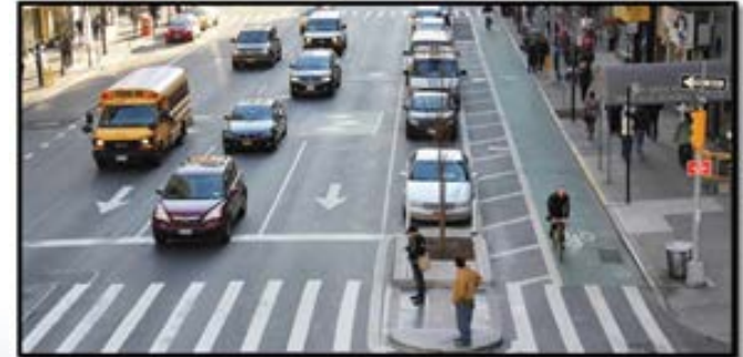
Pedestrian refuge incorporated with protected bike lane
