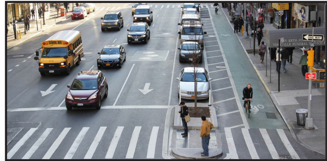
Pedestrian refuge incorporated with protected bike lane
