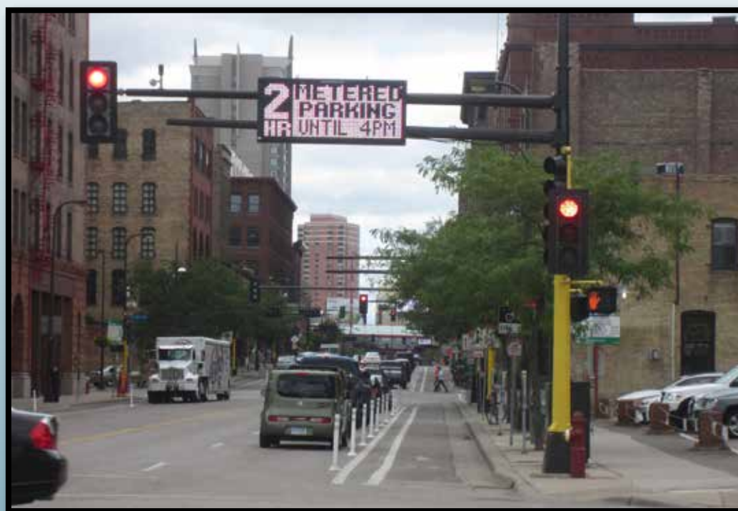
Flexible traffic posts and parking separation
